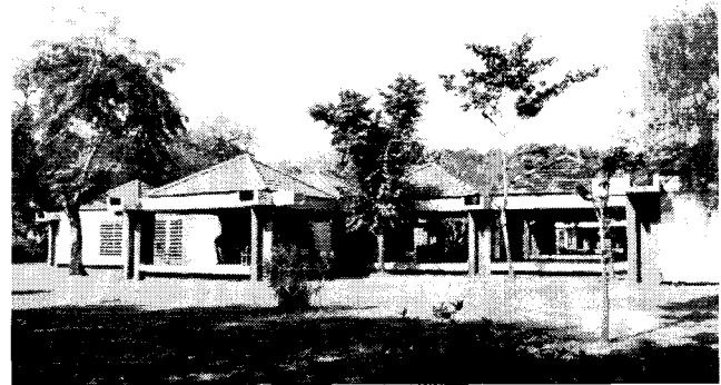
Fig. 4. View from the river side.
